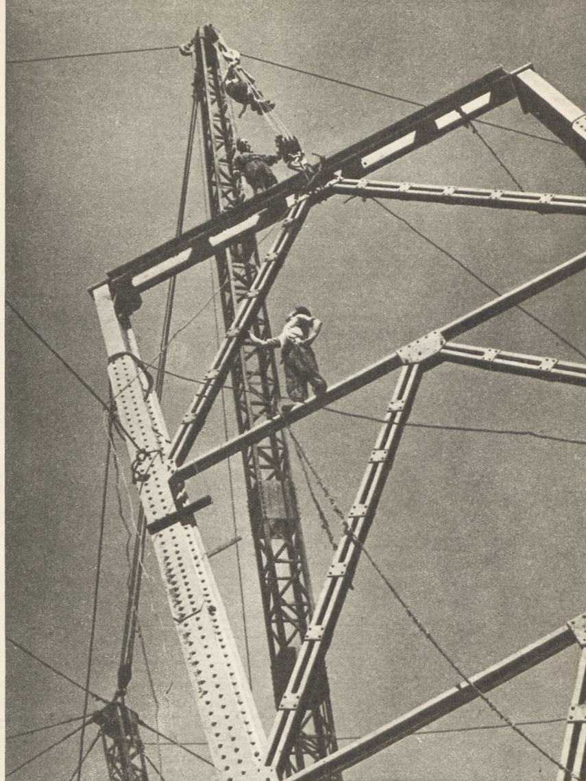
The spectacular rate of increase in industrial and agricultural output during the first half of 1952 was, as in previous years, the outcome of a formidable investment plan. Recent investments include new and large industrial plants, transport services, municipal buildings and housing accomodation. Illustrated: an aerial ropeway in course of erection in the Walbrzych mining centre
