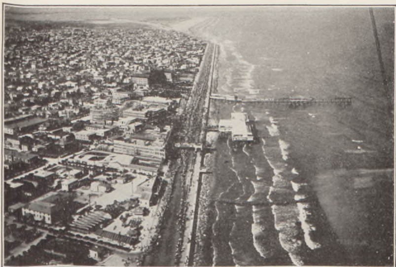
B. PART OF GALVESTON, TEX. General view from an airplane. Shows the sea wall.
