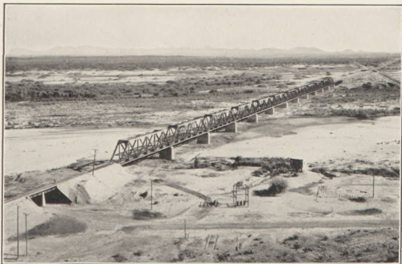
B. VIEW NORTHWARD ACROSS THE GILA RIVER FROM ANTELOPE HILL, BETWEEN WELLTON AND ROLLS, ARIZ.
