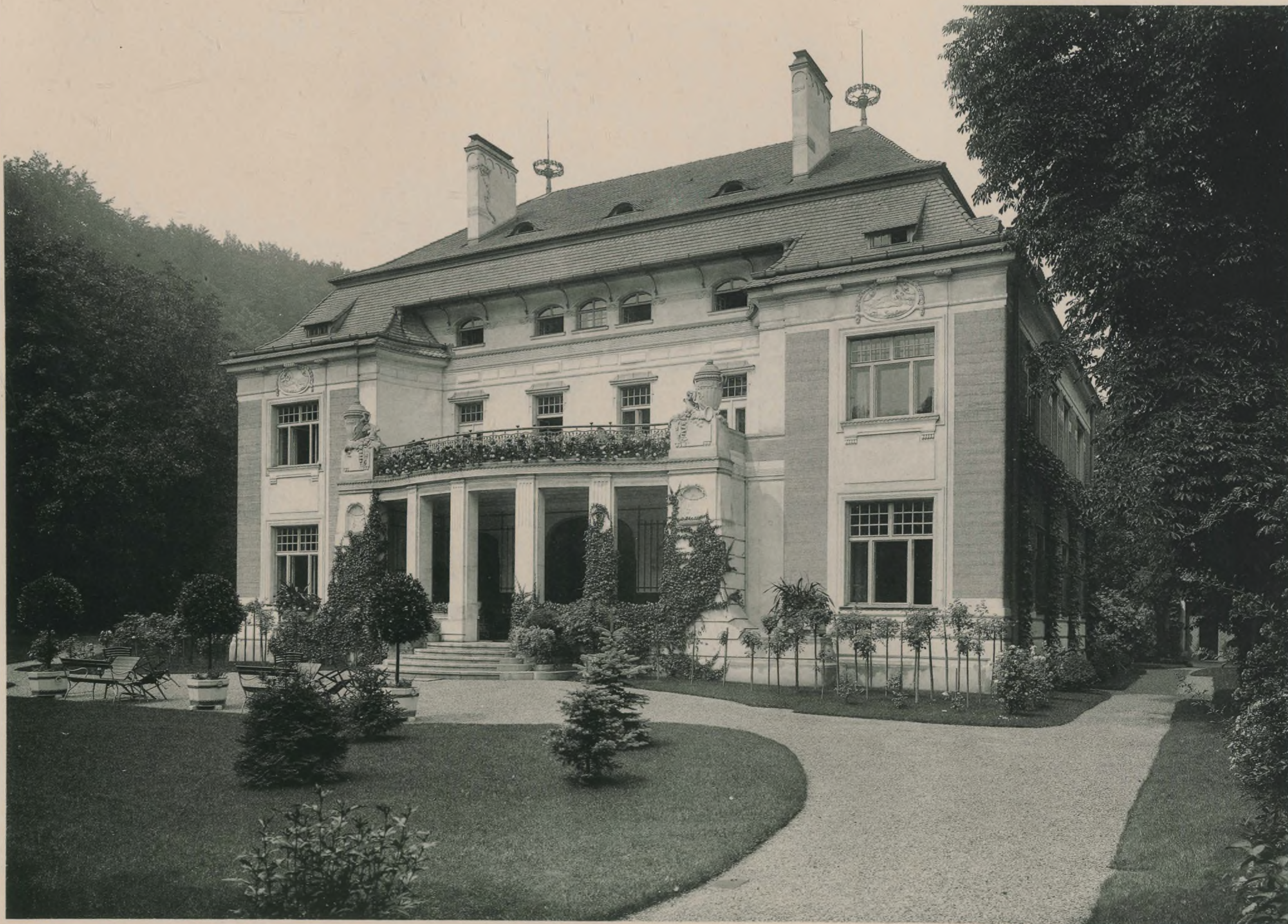
Josel Hackhofer & Fritz Rumpelmayer Arch.
