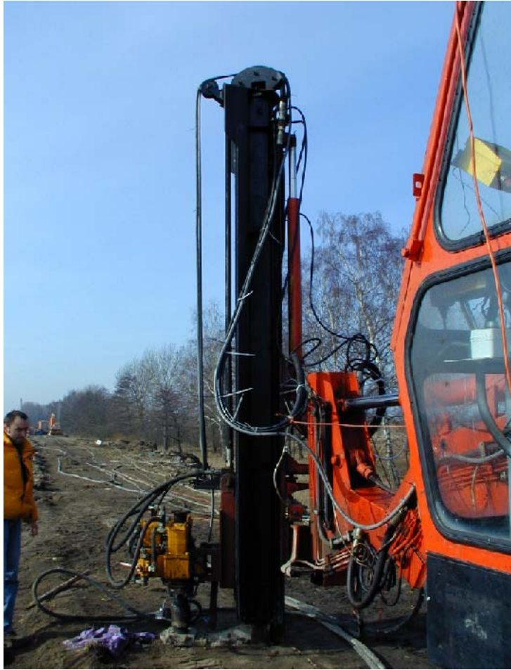
Fig. 1. The drilling rig
