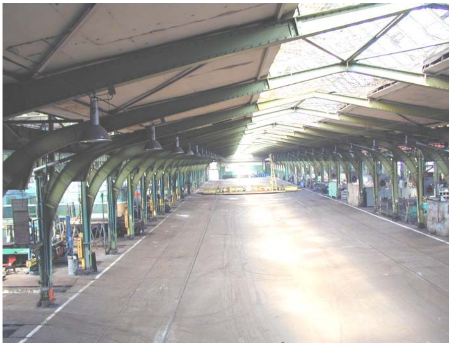
Fig. 1. Main hall of ZNTKiM
