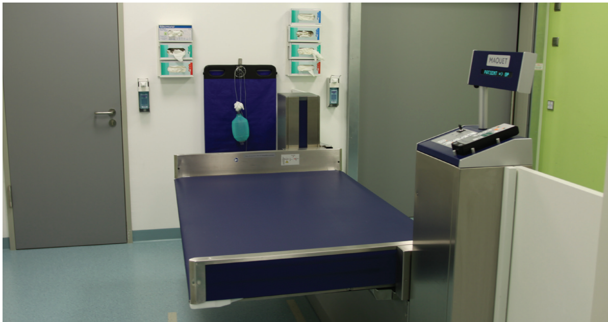
Photograph 6.4 A patient transfer station (in Poland it is assumed that a patient bed should not enter the area of an operating suite); photographed by the Author 2016
