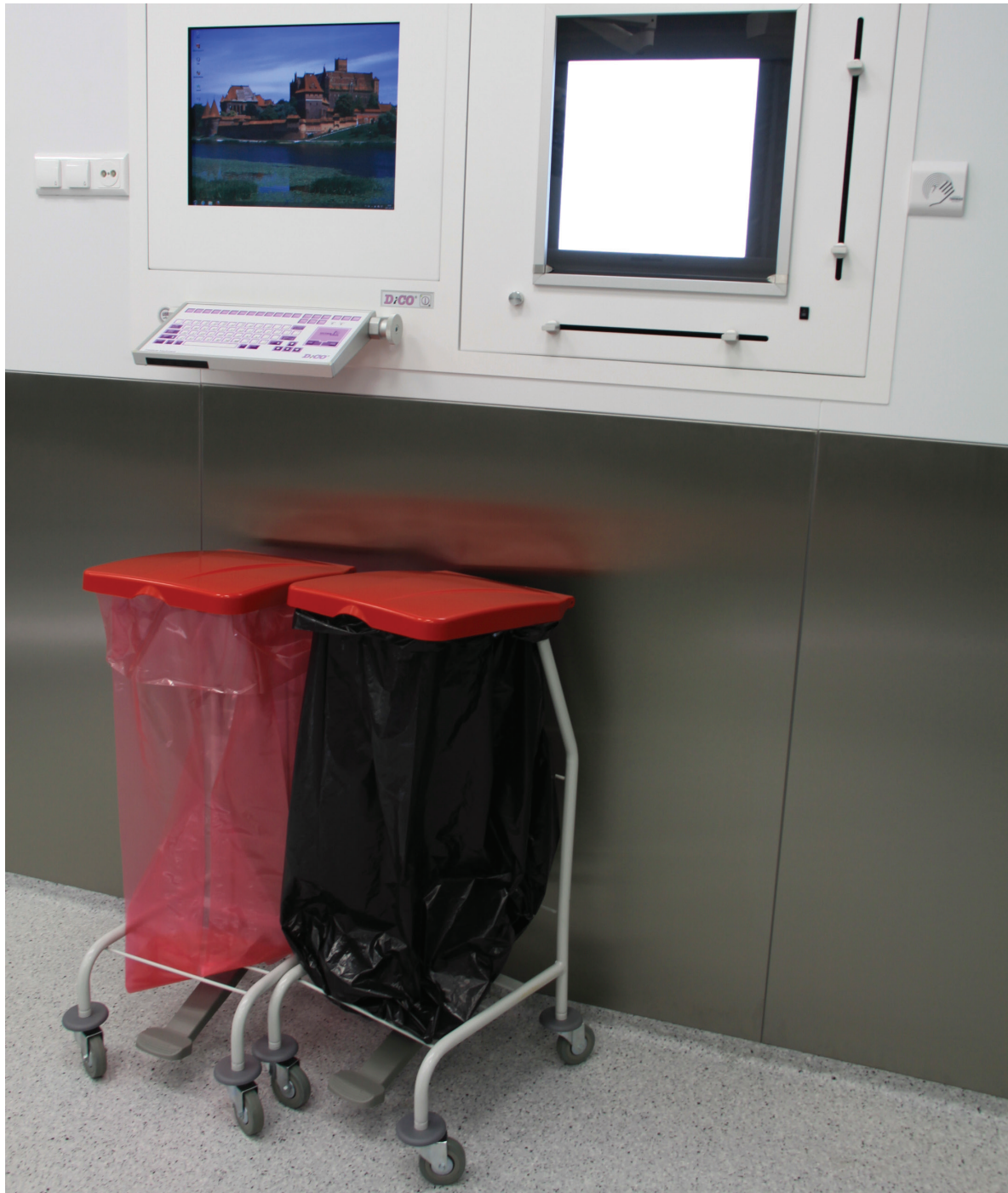
Photograph 6.3.2.4 A display screen with a keyboard in the operating theatre (the elements of the equipment are made in a way that allows for systematic disinfection procedures); photographed by the Author
