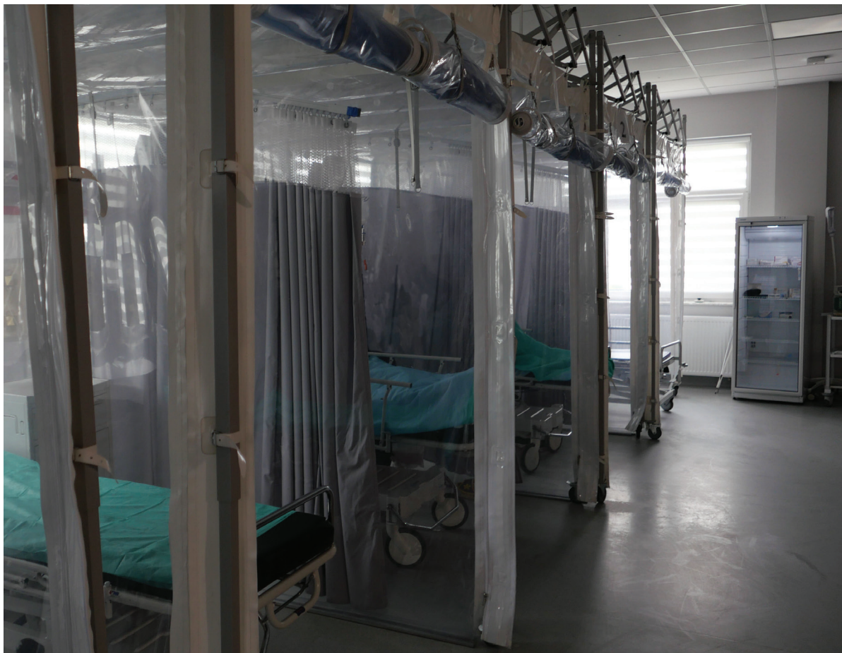
Photograph 4.1.3 Medical care stations at a hospital emergency unit – the implementation of temporary boxes as a solution applied to reduce transmission of infections among patients (the COVID-19 pandemic); photographed by the Author, 2022
