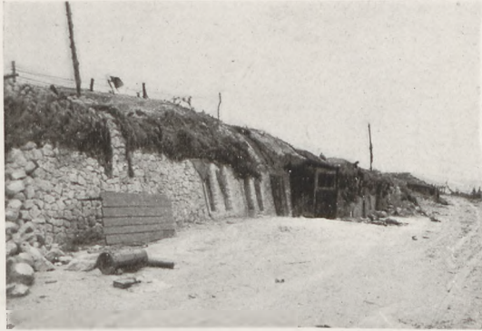
ROAD FROM LOUVE-MONT TO ORNES (Farthest point acces- sible to motor-cars in May, 1919)
