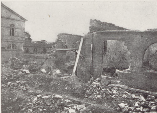
THE CITADEL BUILDINGS AFTER THE BOMBARD- MENTS OF 1916
