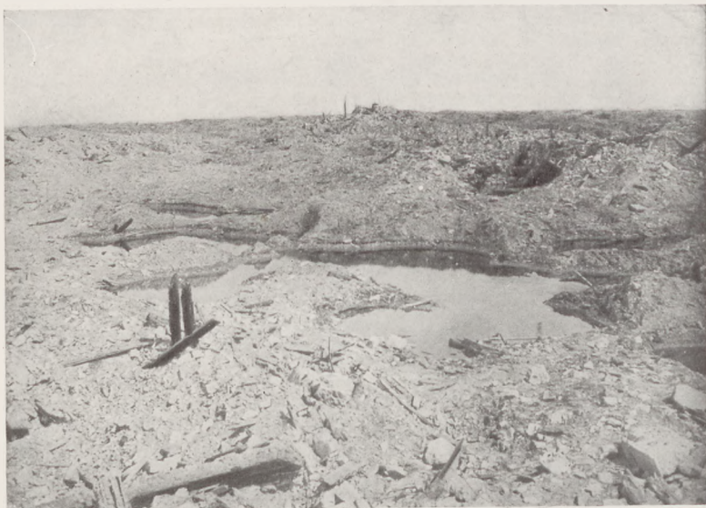
WHERE VAUX VILLAGE ( entirely destroyed ) STOOD BEFORE THE WAR. ( Photo, April 26th, 1917. )
