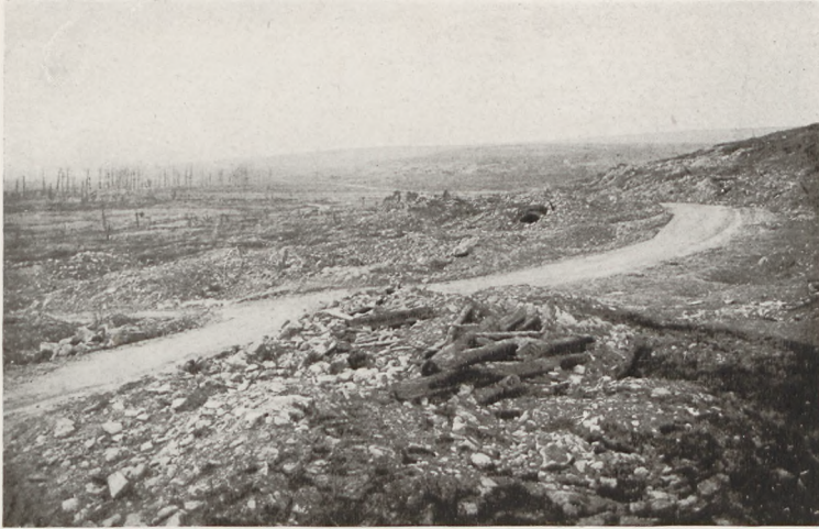
THE CENTRE OF SAMOGNEUX VILLAGE ON THE N. 46, IN MAY, 1919. The village was entirely levelled.
