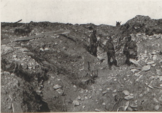
TRENCH ON HILL 304.
