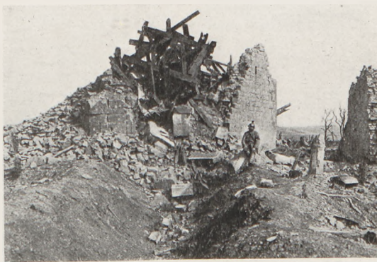
RUINS OF BRAS CHURCH, WHOSE TOWER COLLAPSED. (Photographed in April, 1917)
