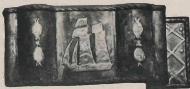
PORTION OF RAIN-WATER HEAD
