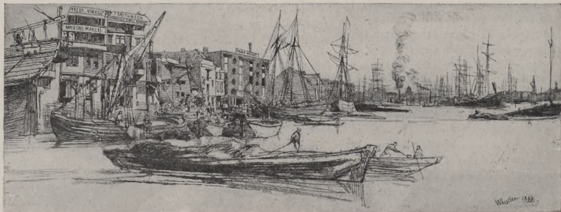
ETCHING: "THAMES WAREHOUSES" (By permission of Frederick Keppel, Esq.)
