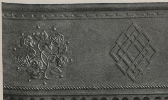
PORTION OF LEAD PARAPETTING
