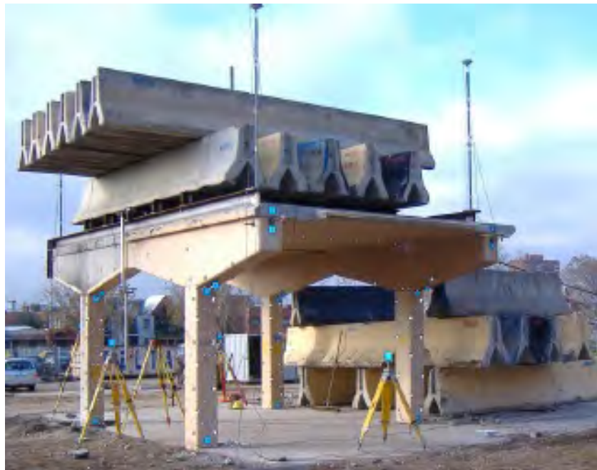
Fig. 2.9: The setup of a push-over test on a part of existing building (Wibowo et al. 2010)
