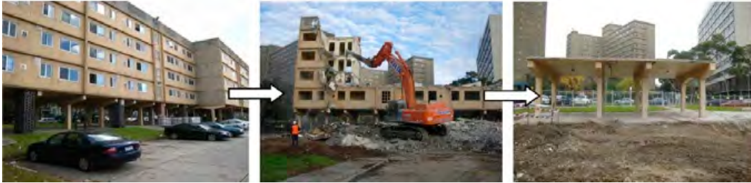
Fig. 2.8: Preparation of a part of existing building for a push-over test (Wibowo et al. 2010)
