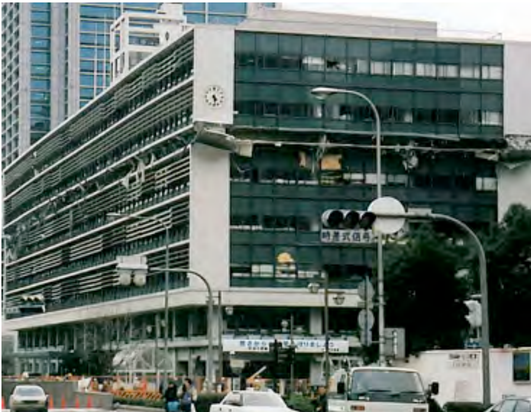
Fig. 1.2: Soft-storey failure of the intermediate storey of building (Kobe earthquake, 1995)
