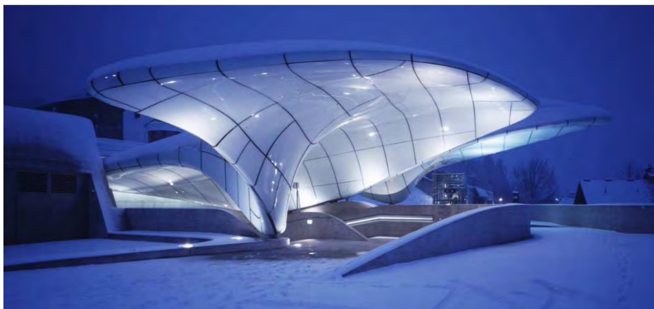
il. 15. Zaha Hadid, Nordpark Railway Stations, Innsbruck, 2007. Hungerburg Station, fotografia: Werner Huthmacher
