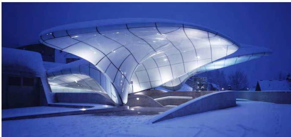
il. 1, Zaha Hadid, Nordpark Railway Stations, Innsbruck, 2007, Hungerburg Station, fotografia: Werner Huthmacher.
