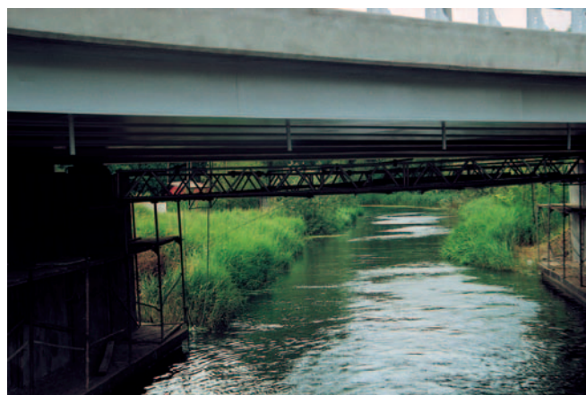
Photo 5. (J. Kulczyk, R. Werszko) A repair of the road bridge over the Upper Noteć Canal. The changes being introduced during the repair work are expected rather to remove the existing obstacles for ship traffic than to cause more troubles .
