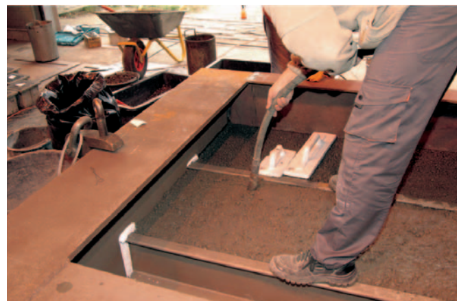
Fig. 3. Application of the concrete into the ship bottom structure
