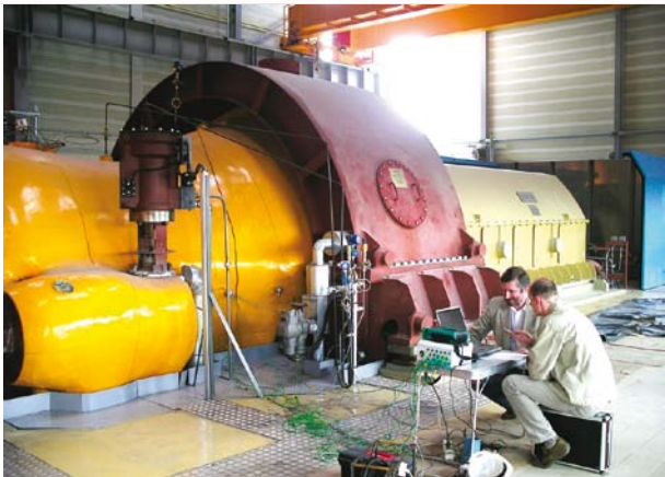
Fig.9 Photo and axial cross-section of 7CK-65 steam turbine set, [4].
