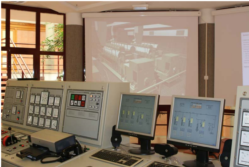
Fig. 3 MED3DH Engine Room Simulator - Main engine's control consoles
