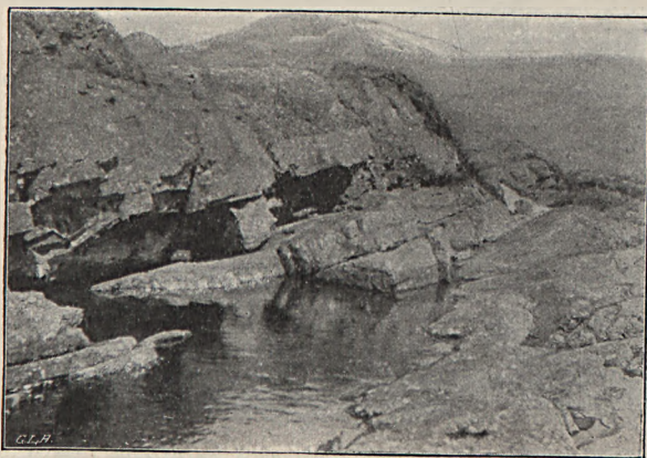
Underminerade sandstenslager i v. Dübens fall. 9/8 98.
