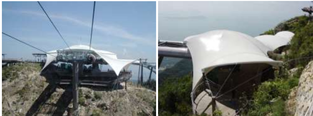
Fig. 1.5. Cableway station, Malaysia ([109])
