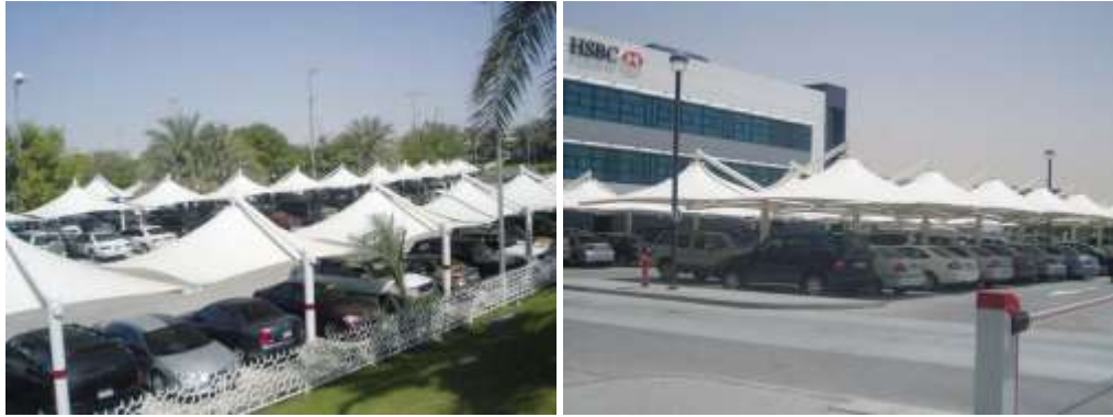
Fig. 1.4. Car park covers, UAE ([109])
