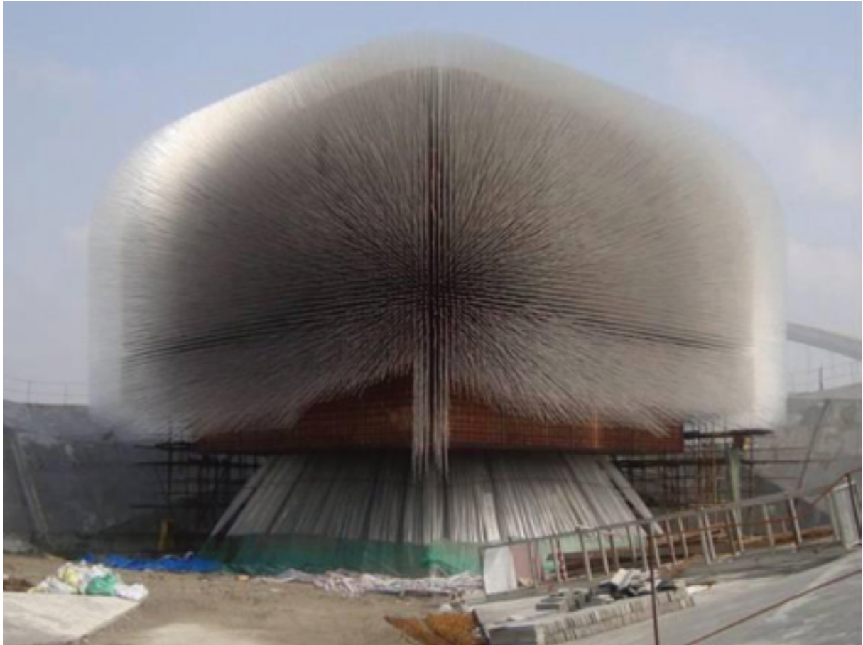
„UK Pavilion at the EXPO 2010“ Shanghai, Heatherwick Studio
