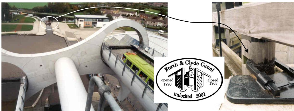
**Fig. 86.** Output of the Falkirk Wheel in Scotland (left) and a top hinge of the gate to it (right)
