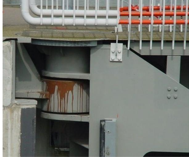
**Fig. 13.** Aesthetically well shaped but difficult to maintain top hinge of the Orange Locks gates in Amsterdam
