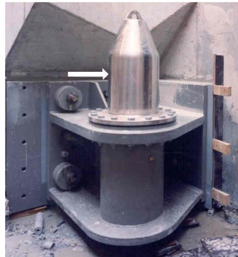
In this case, the problem of collar ring wear has successfully been solved. The hinge is entirely maintenance free and ecologically favorable, as it requires no lubrication. This is particularly important due to the submerged location which limits the inspection and maintenance possibilities. The diameter and height of the ring are large and comparable to the dimensions from Fig. 48, which keeps the contact pressure low – in this case under  $30 \text{ N/mm}^2$ .
