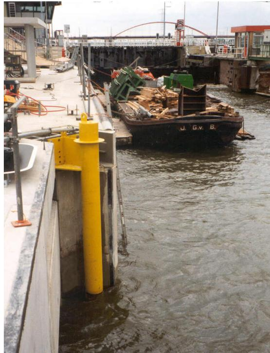
**Fig. 10.** Auxiliary structure for positioning and grouting gate hinge supports
