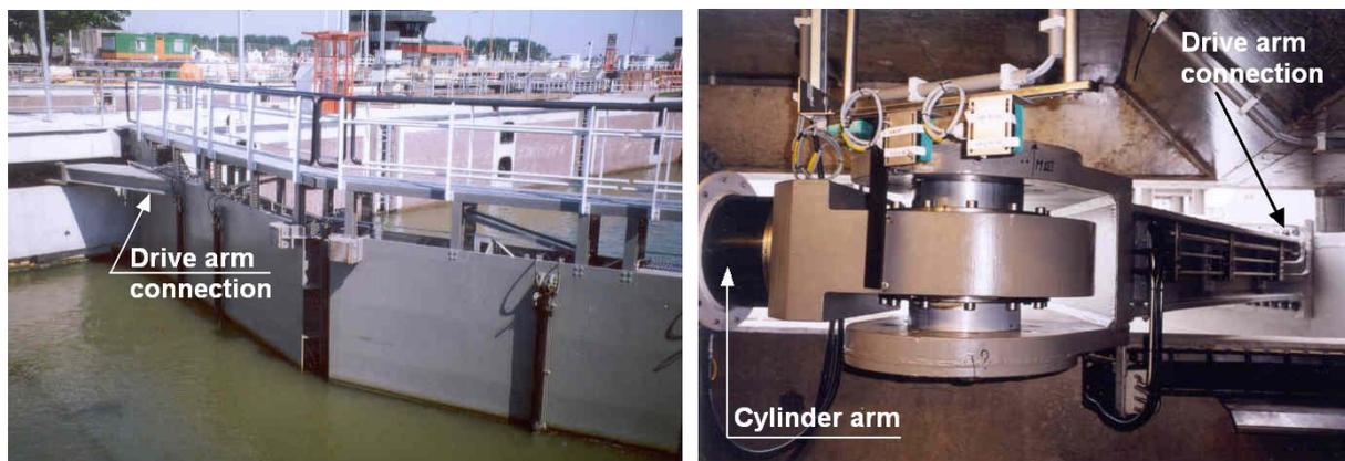
**Fig. 71.** One of the Orange Locks gates (left) and its drive connection (right)
