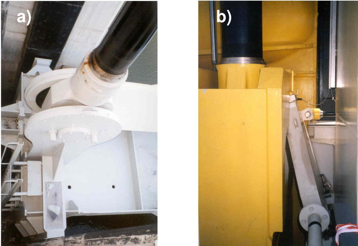
**Fig. 6.** Own weight support of the vertical lift gates:
