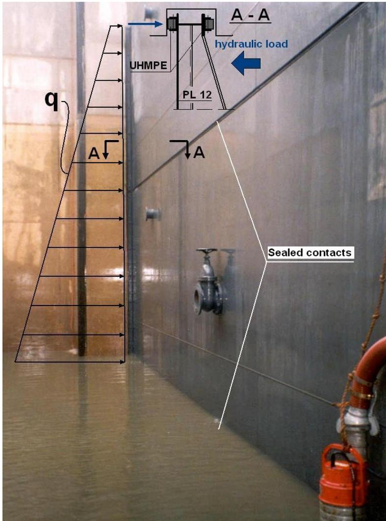
however, not been sealed although the slot surfaces are bare concrete. At the moment when this photo was taken, the hydraulic load on the other side was about 4.50 m of water column. Yet, no leakage can be observed. This is achieved by deliberately allowing for inelastic deformations of polyethylene contact lining, see detail drawn up on the photograph. As result, the material follows all irregularities of the concrete surface, which prevents the leakage [61].
