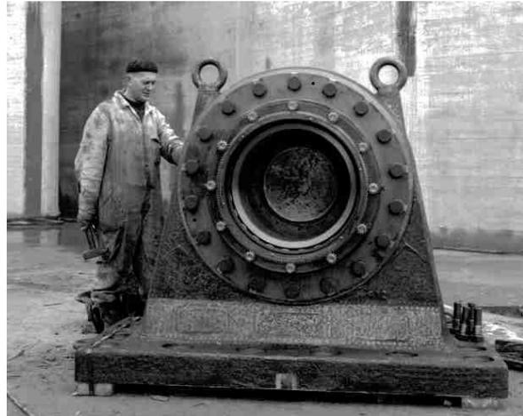
**Fig. 101.** Bearing of the Rhine weir visor gate in Hagestein
