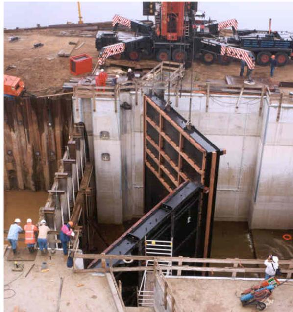
**Fig. 12.** Gate installation in a “dry” chamber by a mobile crane, the Meuse Lock in Lith
