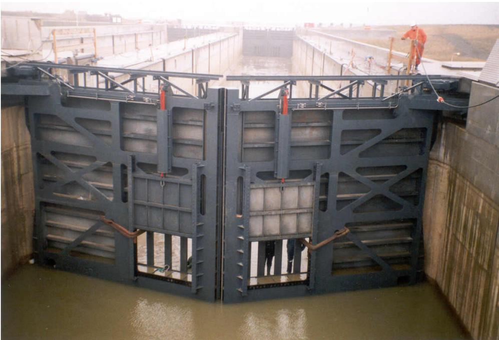
**Fig. 35.** Naviduct Enkhuizen – one of the mitre gates
