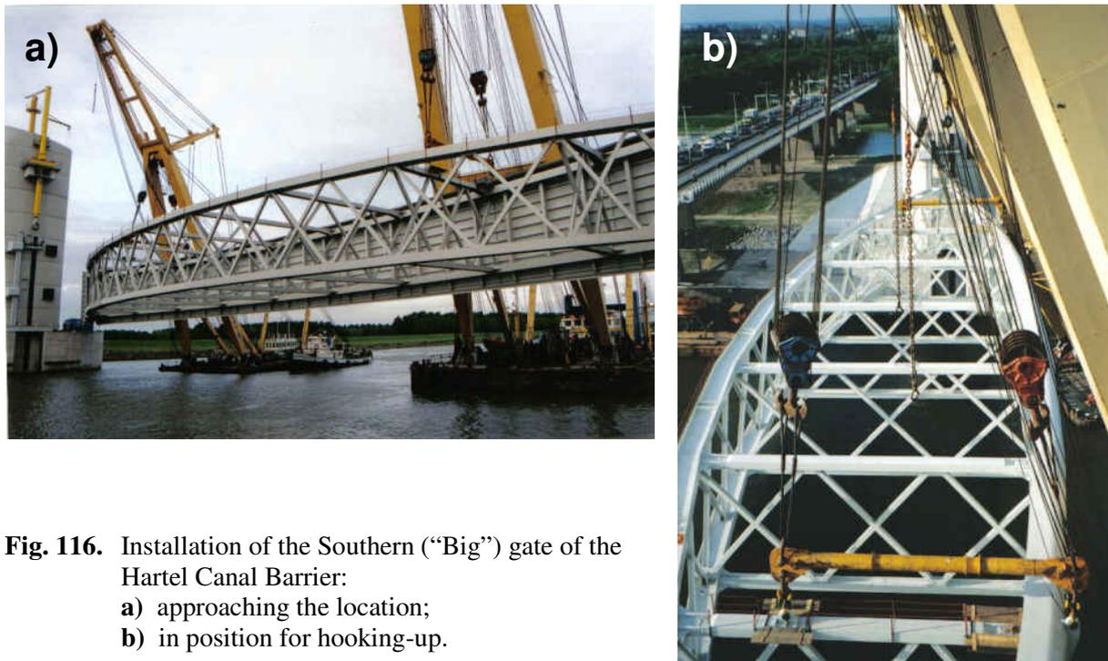
**Fig. 116.** Installation of the Southern (“Big”) gate of the Hartel Canal Barrier:
