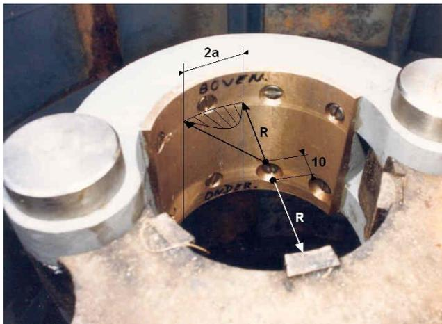
because the horizontal reaction on the ring can only come from the gate own weight. All these gates represent the system of so-called “free” rotation points, in which the hinges do not bear hydraulic loads, see also Fig. 15 in chapter 3. The bronze bushing extends here over an angle of about 120°. The entire gate rotation angle is about 72°. Preserving some margins in boundary positions, we see that the engineer expected the actual contact over an angle of no more than about 30°.
