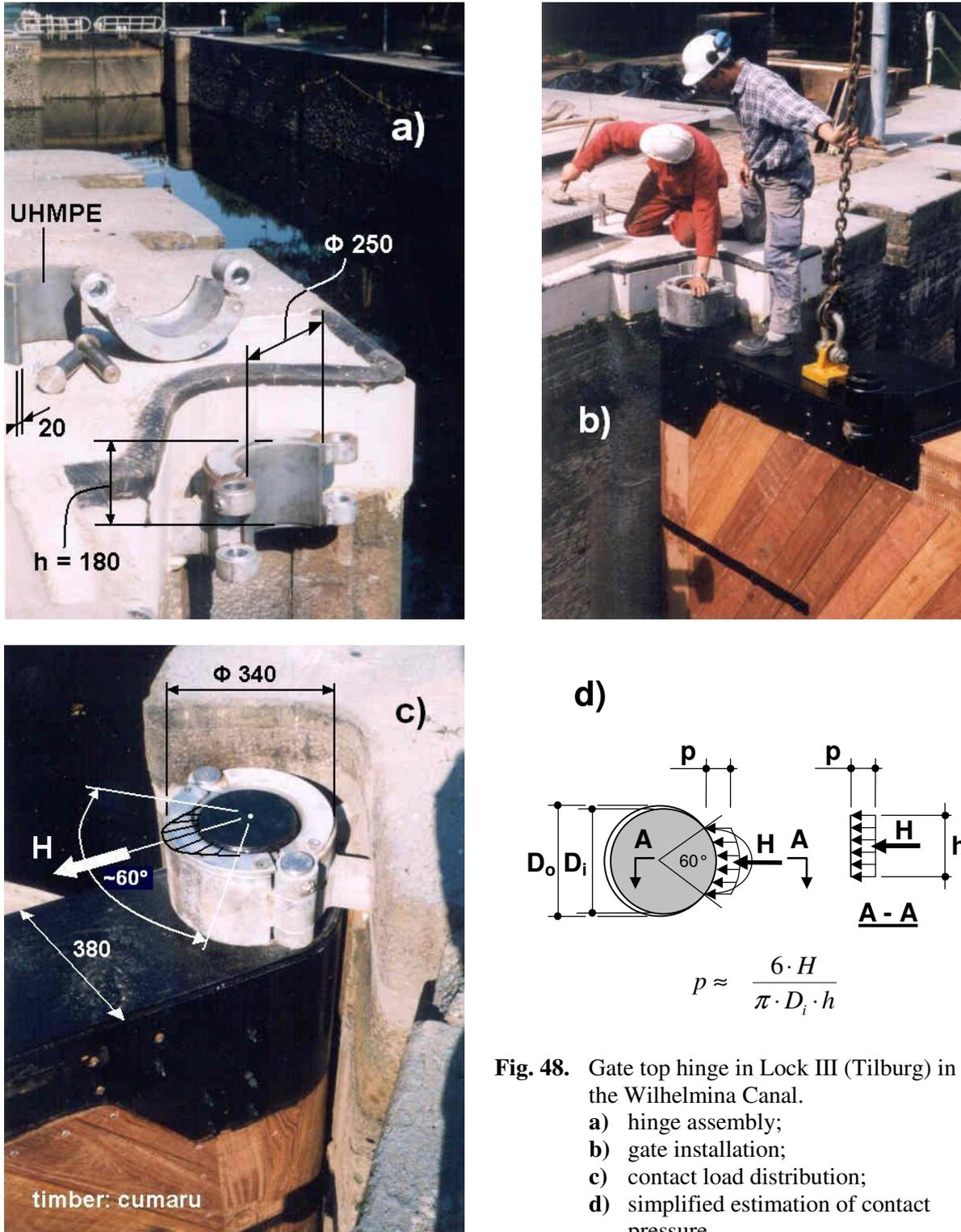
**Fig. 48.** Gate top hinge in Lock III (Tilburg) in the Wilhelmina Canal.
