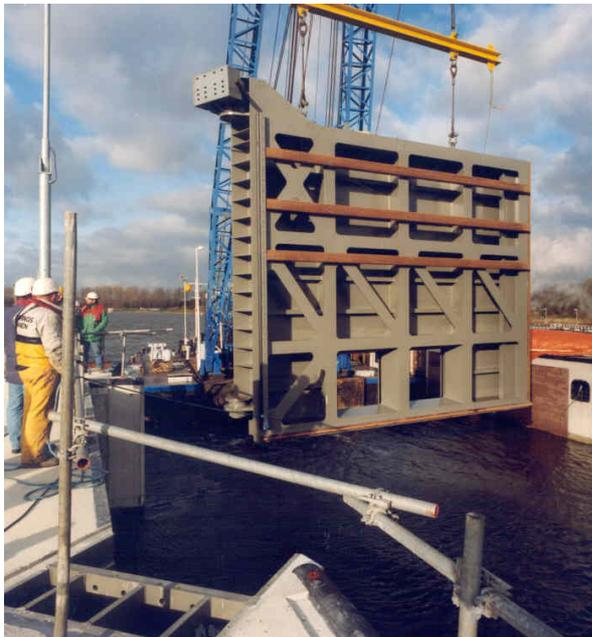
**Fig. 11.** Gate installation in a “wet” chamber by a floating crane, Amsterdam Orange Locks
