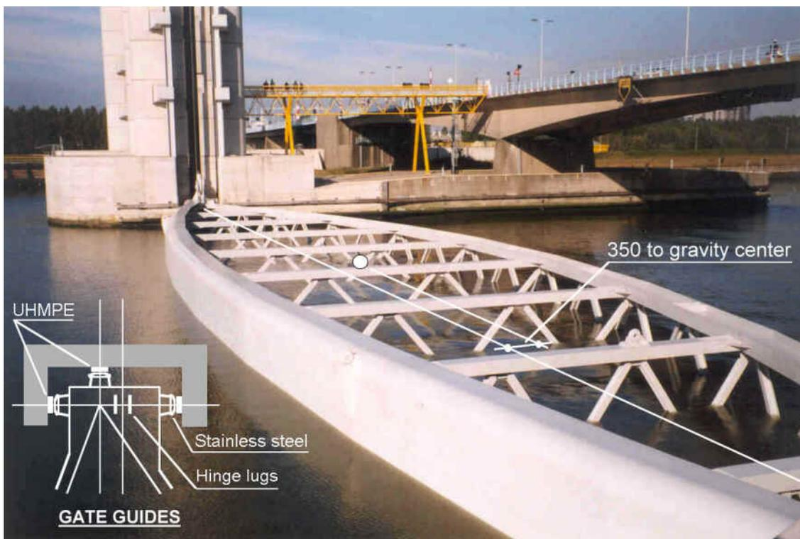
**Fig. 28.** Slide guiding of the Hartel Canal Barrier near Rotterdam
