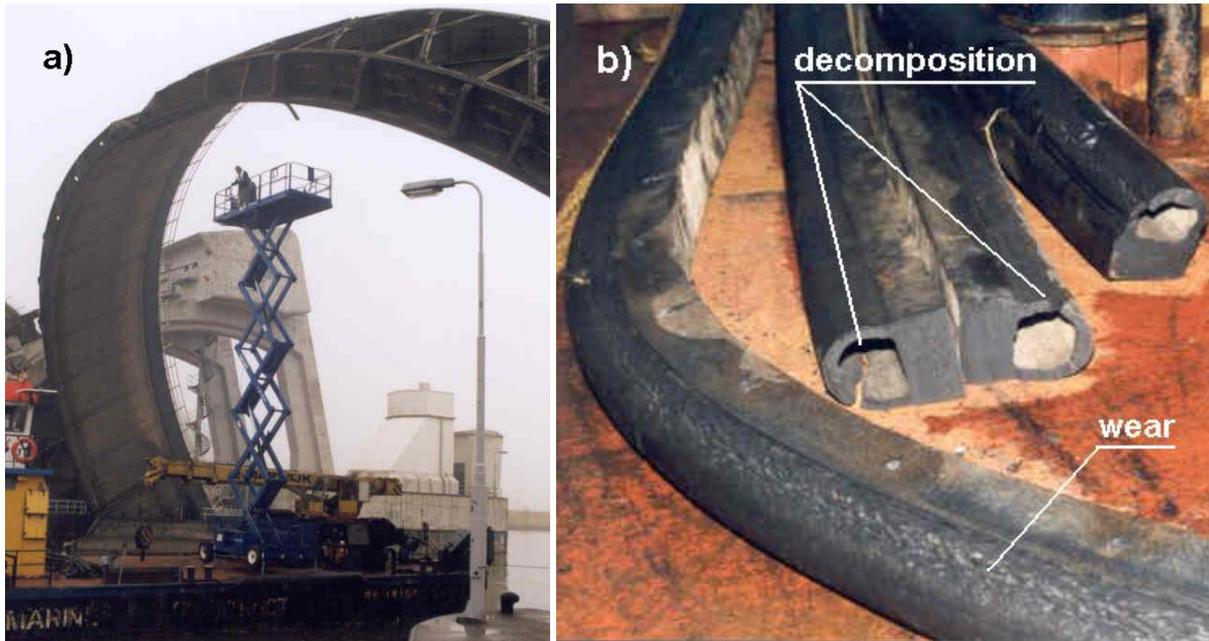
**Fig. 32.** Bottom edge renovation of the Hagestein Weir:
