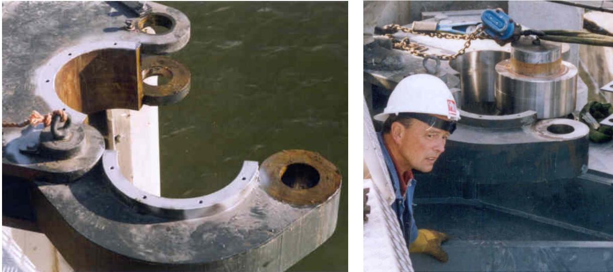
**Fig. 118.** Lockable collar ring of the mitre gates in the Naviduct Enkhuizen
