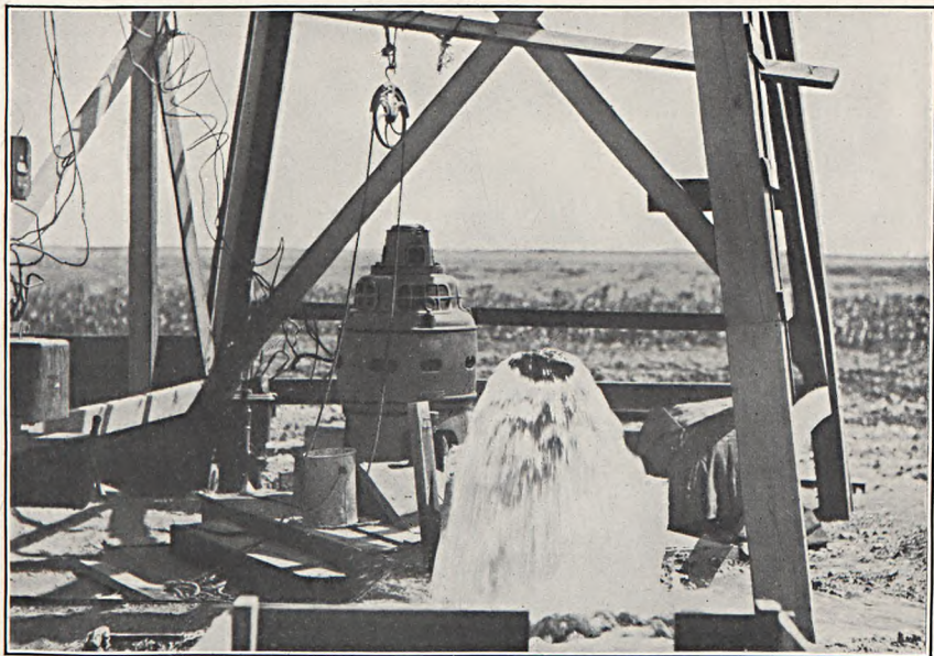
B. WELL ON YOUNG RANCH SOUTHWEST OF DEMING, N. MEX. Pumped by electricity to yield 700 gallons a minute.
