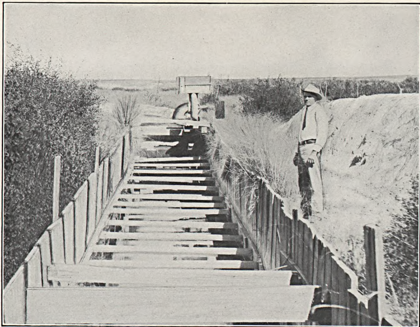
A. DITCH AT SOLIGNAC RANCH, 8 MILES EAST OF DEMING, N. MEX. Dug to surface of underflow.
