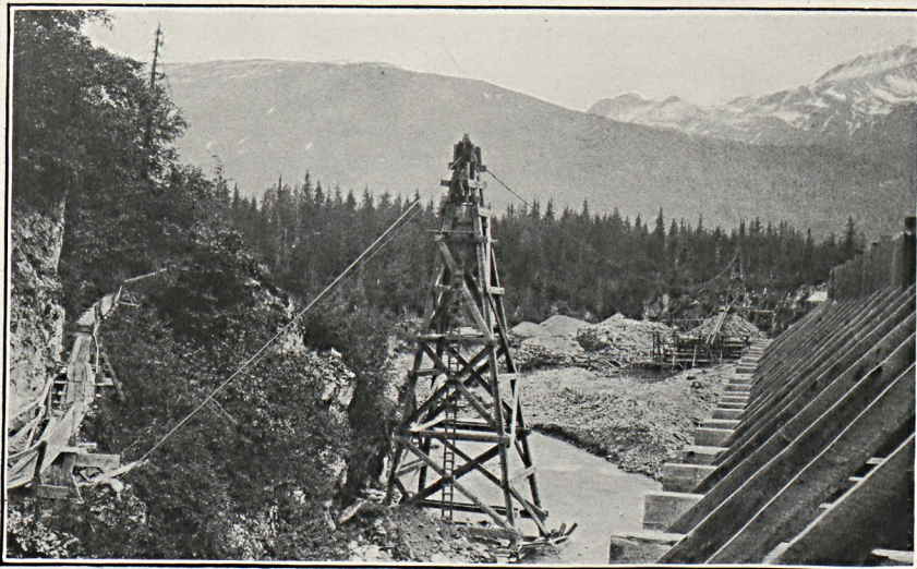
A. CABLE TRAMWAY FORMERLY USED IN STACKING BOULDERS, PORCUPINE CREEK.
