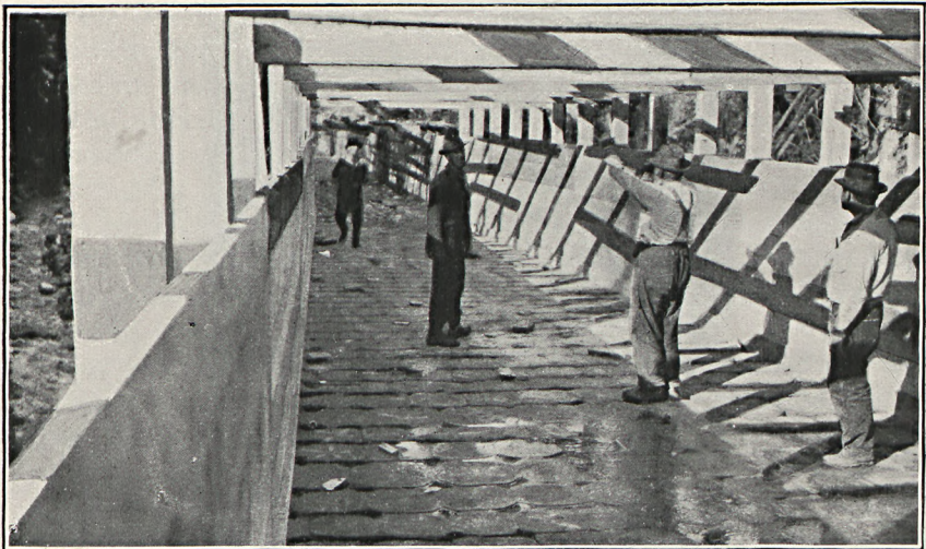
B. DETAIL OF GLACIER CREEK FLUME, SHOWING USE OF RIFFLE BLOCKS.
