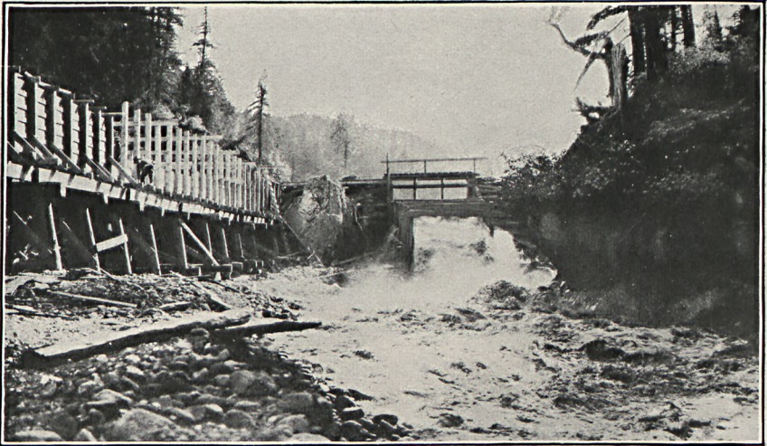
A. FLUME AND SPILLWAY, GLACIER CREEK DAM.
