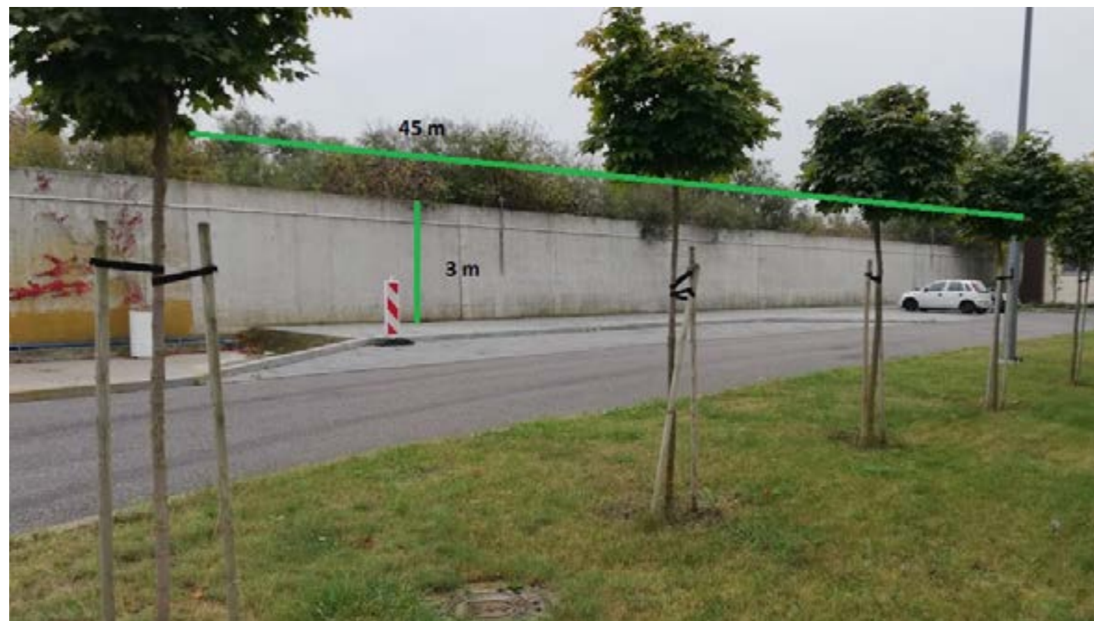
Ryc. 1. Fragmenty muru Il. 1. Wall fragments
