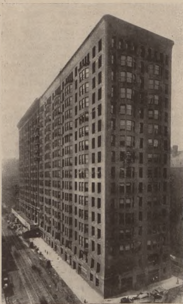
ARCHITEKT: ROOT, MONADNOCK-BLOCK IN CHICAGO
