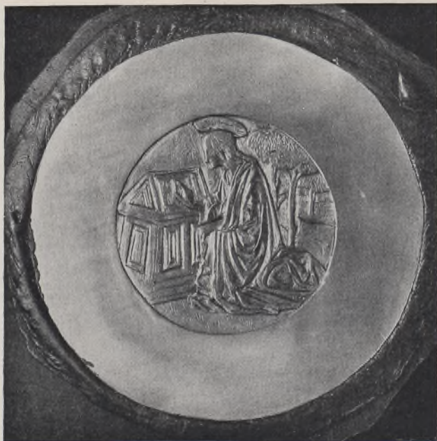
PIECE OF SILVER FIXED ON PITCH BLOCK, SHOWING A FIGURE IN PROCESS OF BEING CARVED FOR BASSETAILLE ENAMEL BY ALEXANDER FISHER
