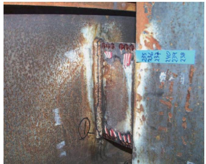
Fig. 5. Example of fatigue crack in welded joint of ship structure detail [6]
