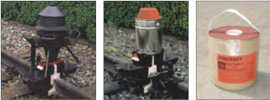
Rys. 7.26. System tygli firmy Elektro-Thermit [38]
