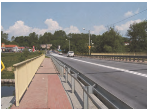
Fig. 3.44. General view of the bridge
