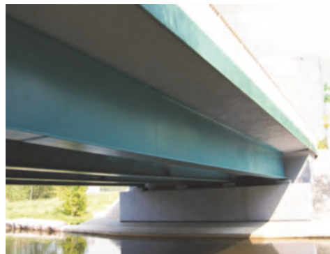
Fig. 3.45. Side view of the bridge
