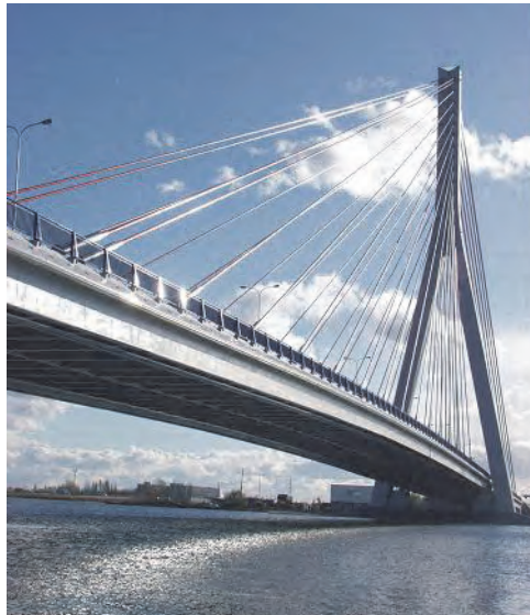
Fig. 2.5. Photo of the bridge over the Vistula River in Gdańsk
